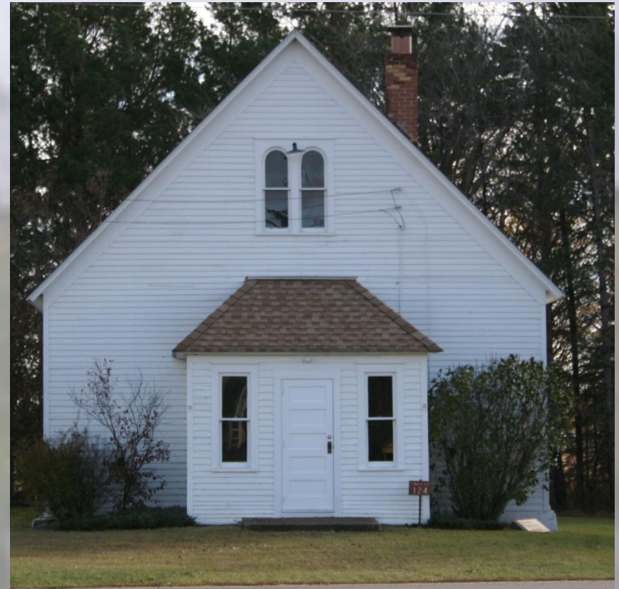
The Temperance Hall at Temperance Corner, north of Cokato on County RD 3
