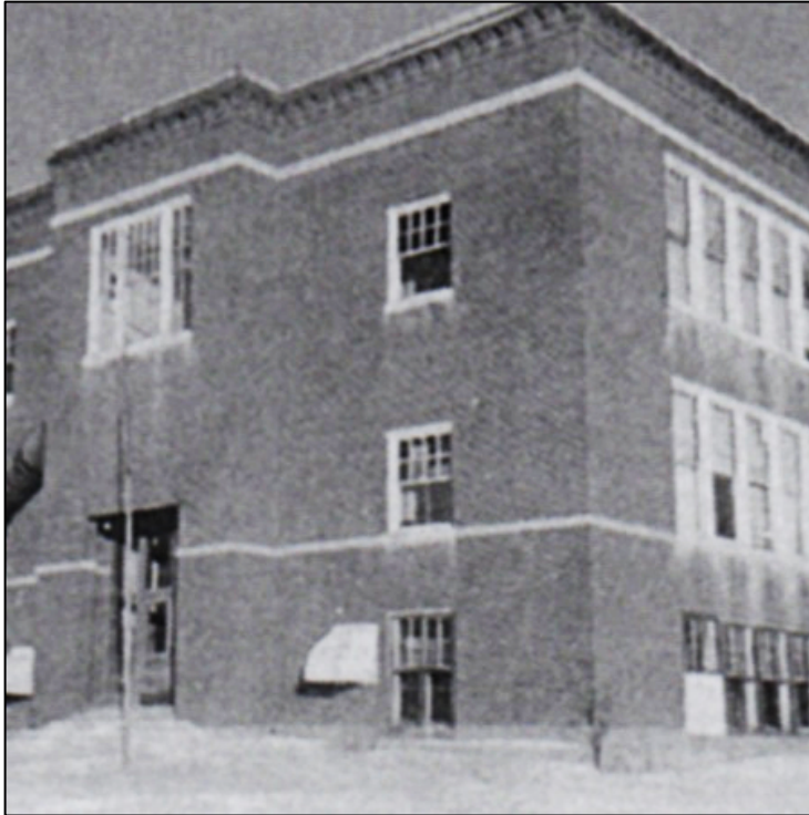
Historic view 5. Undated view of the north end. Note the ventilator hoods flanking the doorway.
